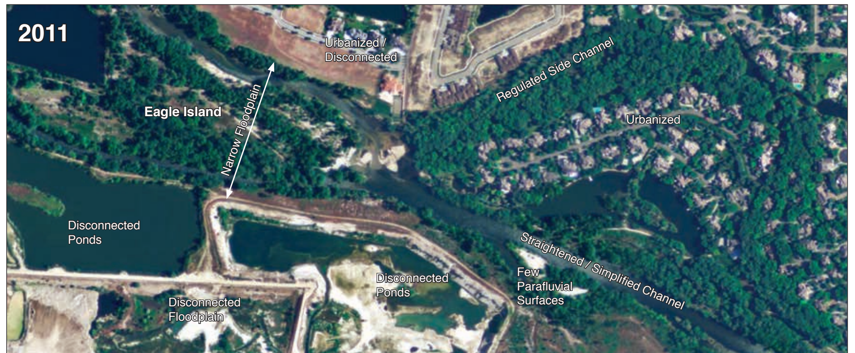
Head of Eagle Island / River Channel 2011: Aerial Image of the Boise River near the head of Eagle Island in 2011, more than 50 years after the completion of Lucky Peak Dam. The river channel is simplified and the floodplain disconnected and confined by urban development and flood control.
