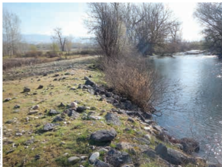
Channel confined by levee and rip-rap. Along much of the Boise River the channel is confined and simplified. Levees and rip-rap are designed to prevent channel migration and confine water to the main channel. The former floodplain is then disconnected from the river. Moving these types of structures back from the main channel and allowing the river to access the existing ground brings multiple benefits, including wetland and riparian development, increased habitat for fish and wildlife, and flood conveyance.
