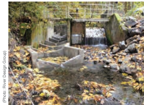
Rock Creek, OR. A fish ladder was constructed to provide fish passage around an irrigation structure.
