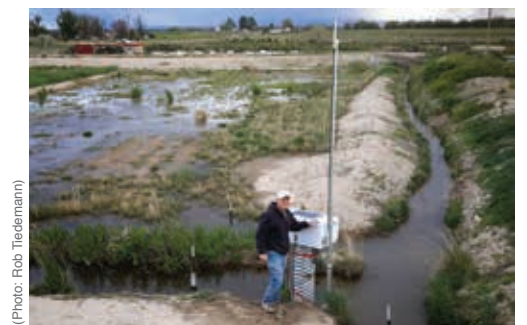
North Alkali Drain Water Quality Improvement Pilot Project, Parma. Implemented in 2014 by Integrated Watershed Solutions, this project tests whether a sedimentation basin in combination with constructed wetlands can remove significant quantities of sediment and phosphorus from irrigation return waters. Initial results show effective removal of both pollutants.
