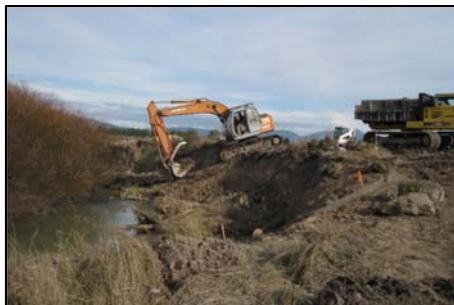
Figure 32. Floodplain excavation on the Reimer reach.
