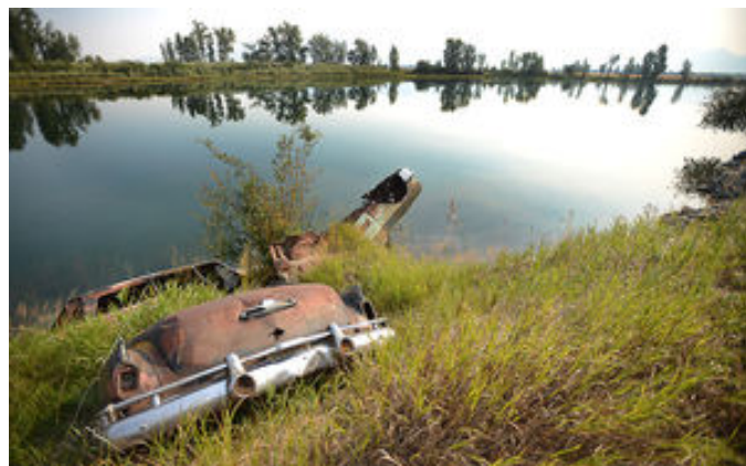
Figure 28. Historical streambank stabilization technique using car bodies on Flathead River near its confluence with the Stillwater River.
