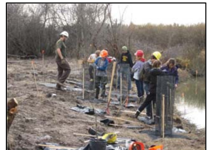
Figure 33. Project FREEFLOW students planting riparian vegetation on excavated floodplain.
