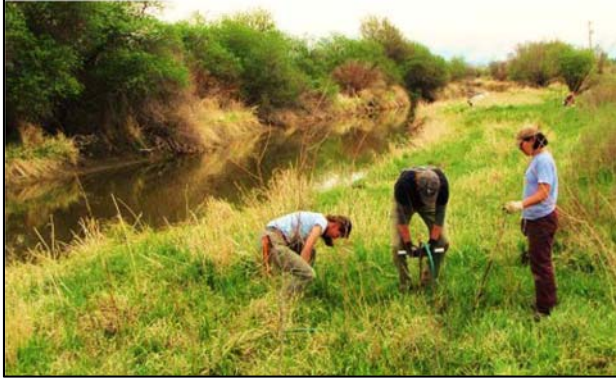
Figure 20. Volunteers planting willow stakes into the ground with water jet stinger.
