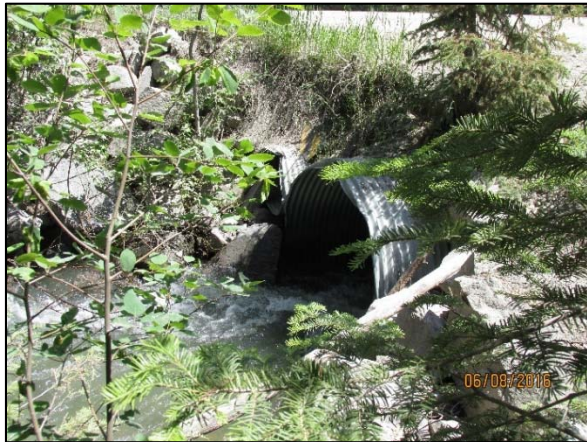
Figure 34. Upstream end of Haskill Basin Rd. culvert.
