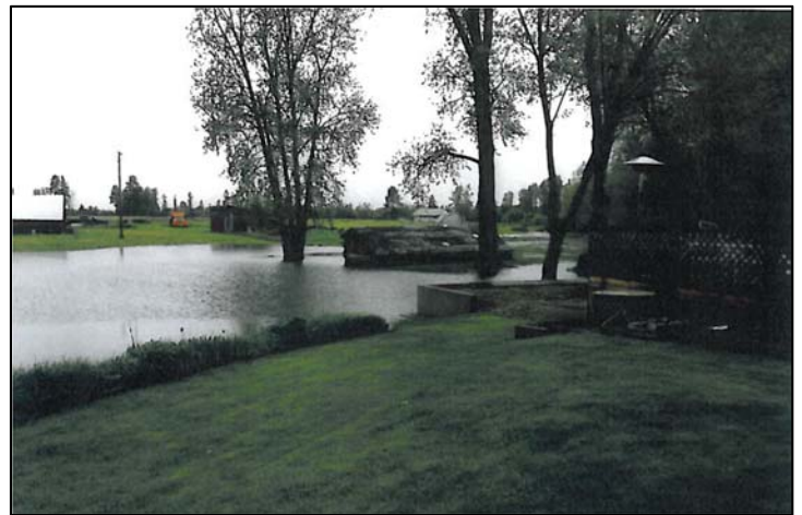
Figure 57. Flooding during spring flow caused by backed-up waters from undersized culverts.
