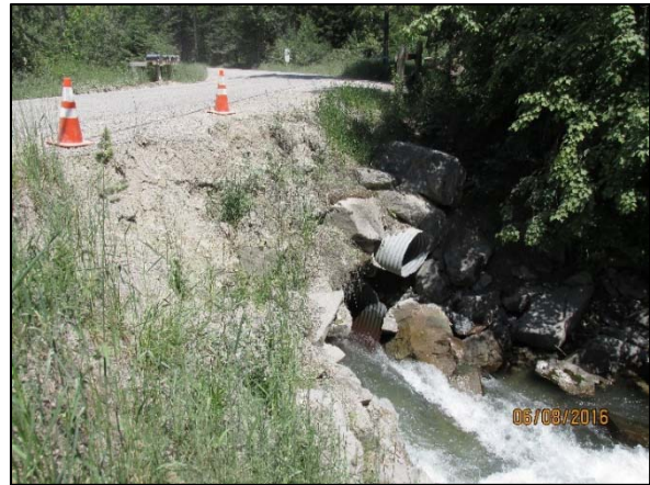
Figure 35. Downstream end of Haskill Basin Rd. culvert.
