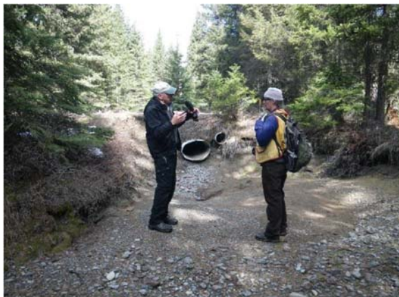
Figure 39. Undersized culvert.
