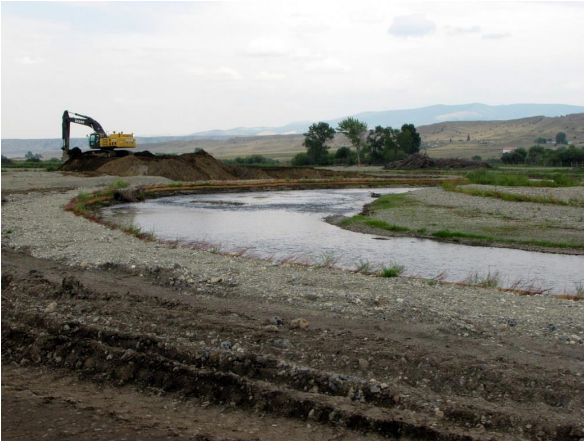
Figure 33- Restoration work underway on the CFC's Dry Cottonwood Creek Ranch in 2015.
