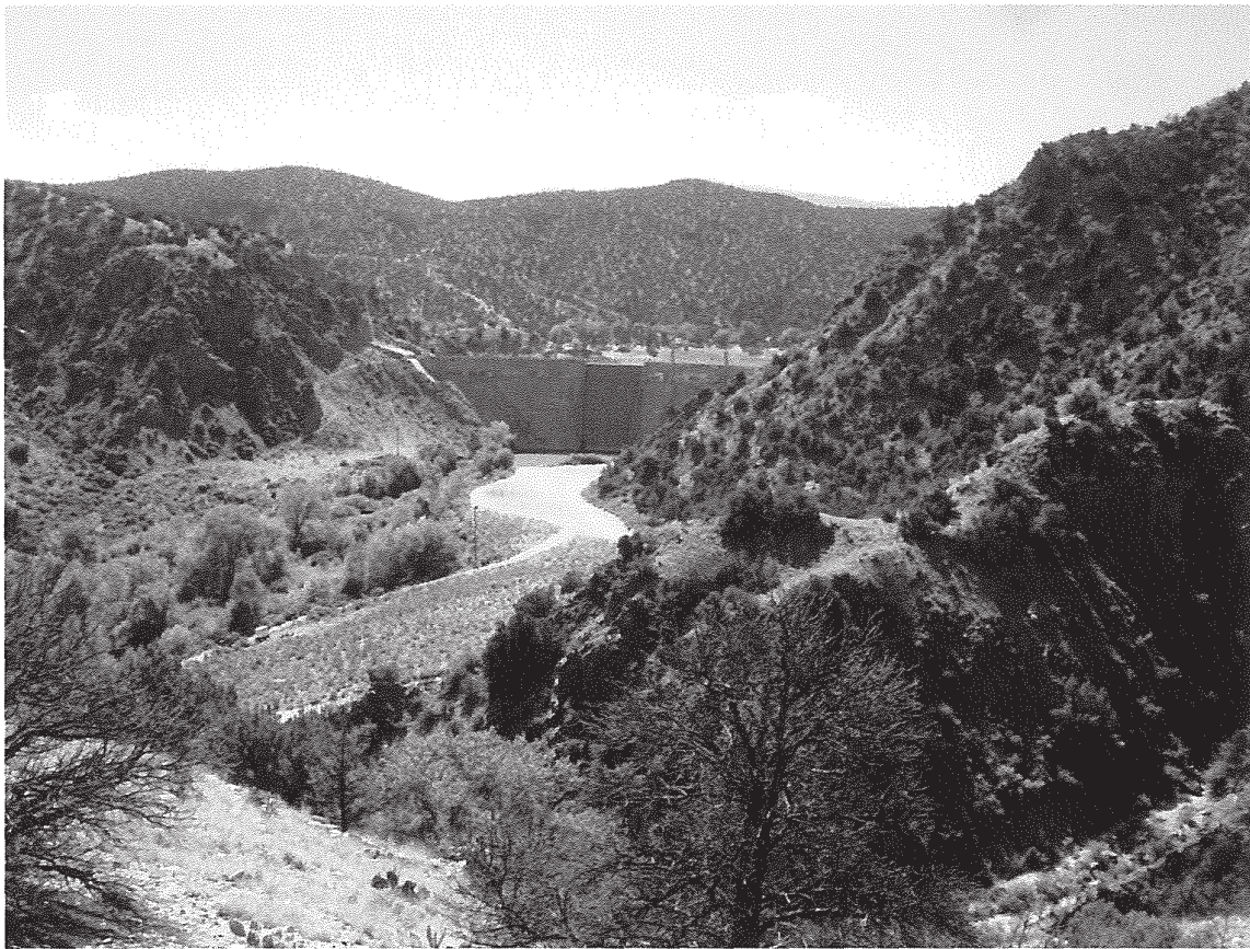
Photograph of Santa Cruz Dam, year 2013.
