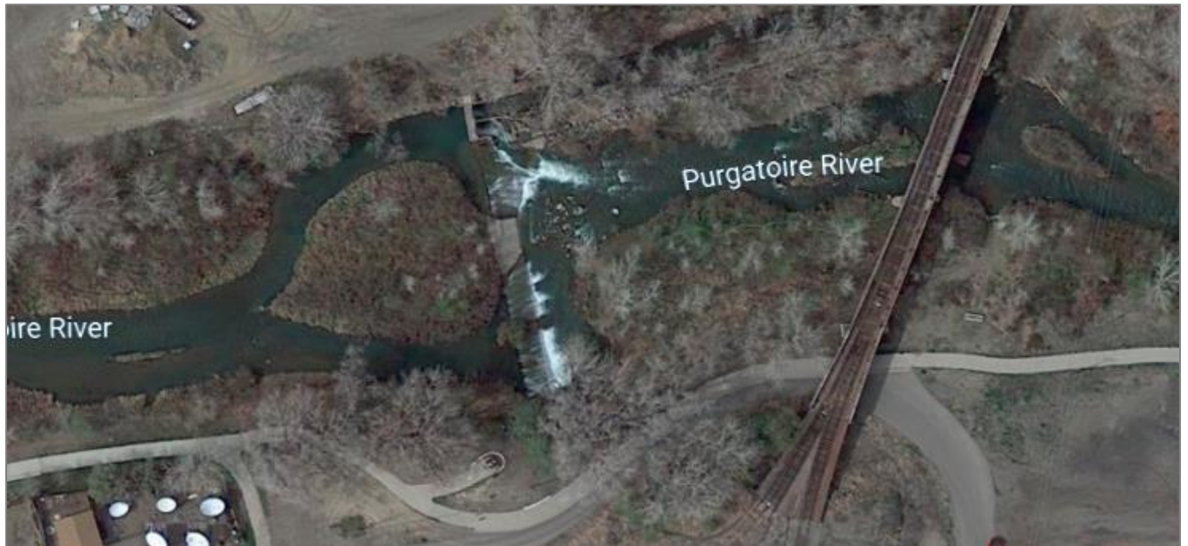
Overhead closeup image of Baca-Picketwire diversion dam, ditch, headgate, and island. The headgate and ditch are on river left (top of photo). The diversion dam stretches across the entire width of the river.
