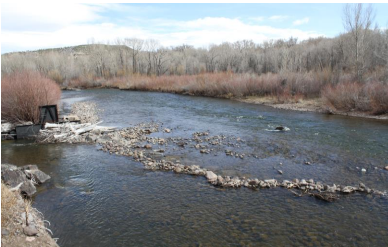
Figure 2: Mecitos Ditch diversion dam on the Conejos River.
