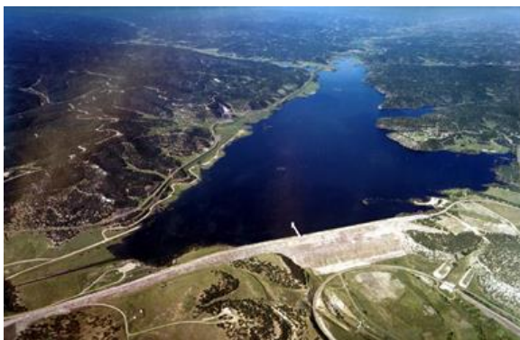
Figure 3: Aerial photo of Trinidad Lake and Trinidad Dam
