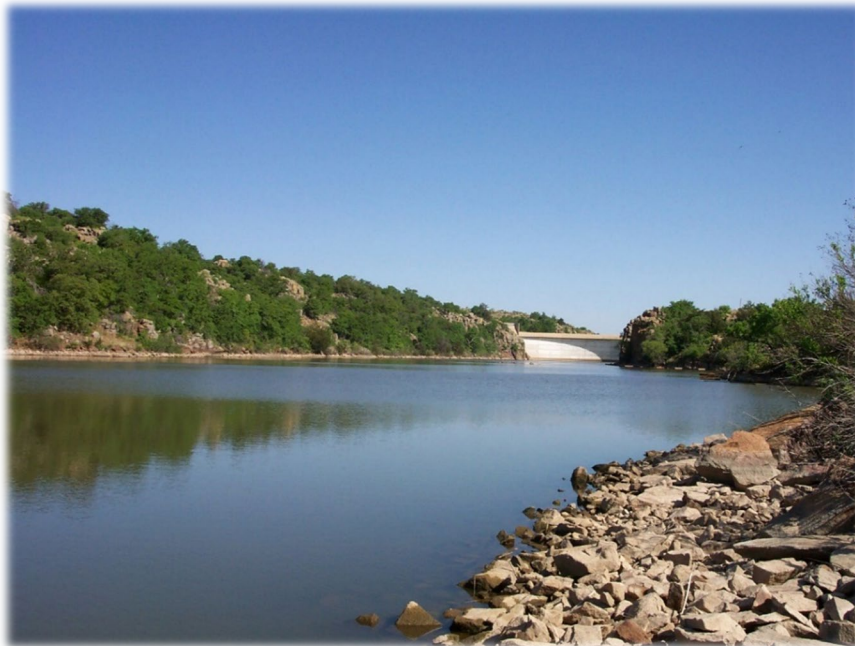
Downstream of Mountain Park Dam, Mountain Park Project.
