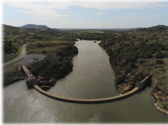
Mountain Park Dam, Tom Steed Reservoir.
