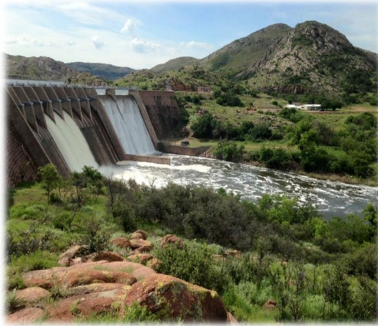
Altus Dam, W.C. Austin Project.
