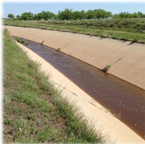
Bretch Canal, Mountain Park Project.
