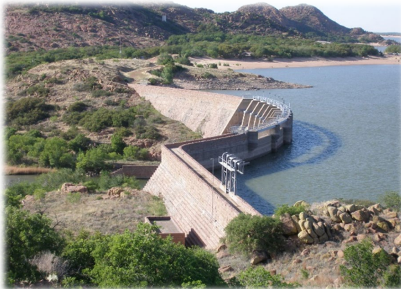
Altus Dam, Lugert-Altus Reservoir.
