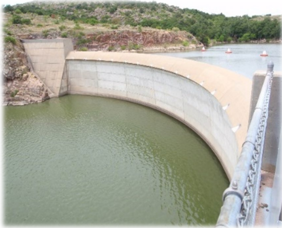
Mountain Park Dam, Mountain Park Project.
