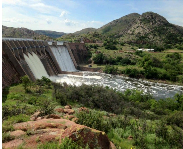
Figure 2. Altus Dam, W.C. Austin Project.
