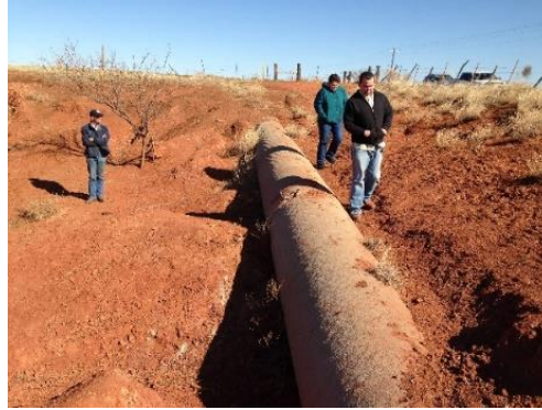
Figure 4. Altus Aqueduct, Mountain Park Project.
