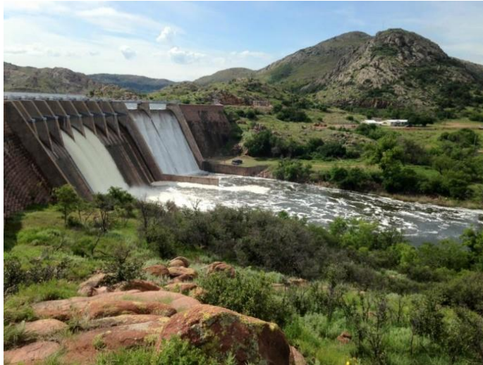
Figure 2. Altus Dam, W.C. Austin Project
