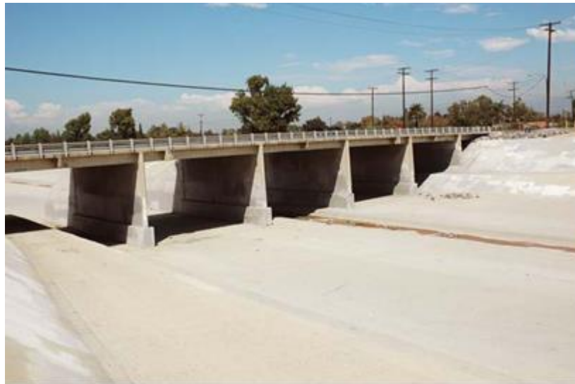
Figure 5: Santa Ana River bridge and channel (Source: http://alamar.sdsu.edu/projectphotosrrr.html )
