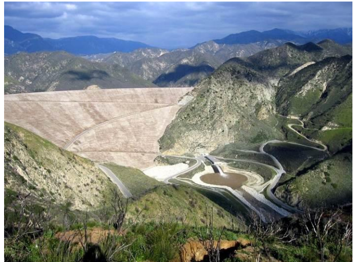
Figure 4: Seven Oaks Dam in the San Jacinto Mountains (Source: http://en.wikipedia.org/wiki/File:Seven_Oaks_Dam.jpg )
