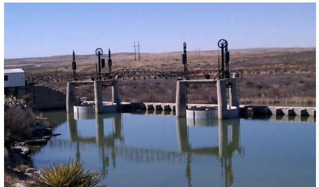
Figure 24. Avalon Dam (Reclamation).
