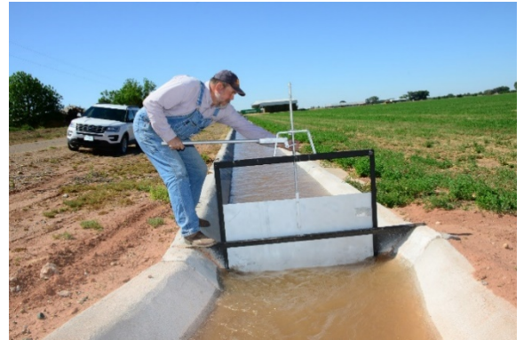
Figure 26. Wade Holdeman, FSID manager, adjusts a sluice gate on an irrigation ditch (Natural Resources Conservation Service [NRCS] Photo by Rey T. Adame, all rights reserved).
