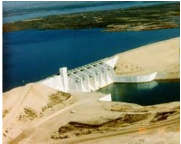
Figure 23. Brantley Dam (Reclamation).
