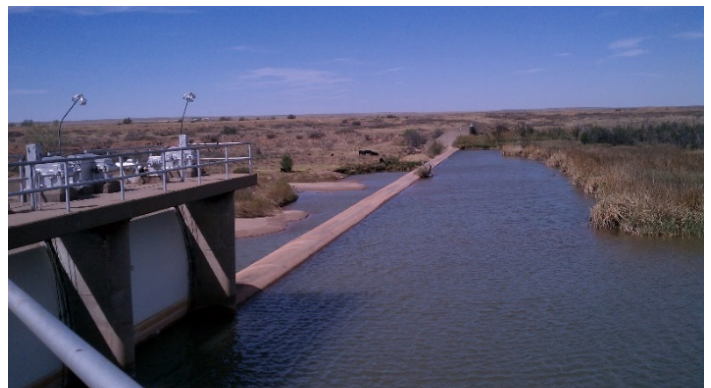
Figure 22. Fort Sumner Diversion Dam (Reclamation).
