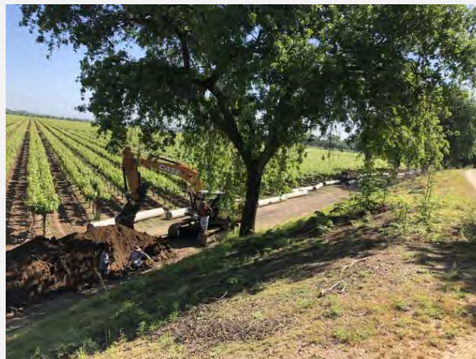
Figure 5: Construction at the on-farm recharge site.
