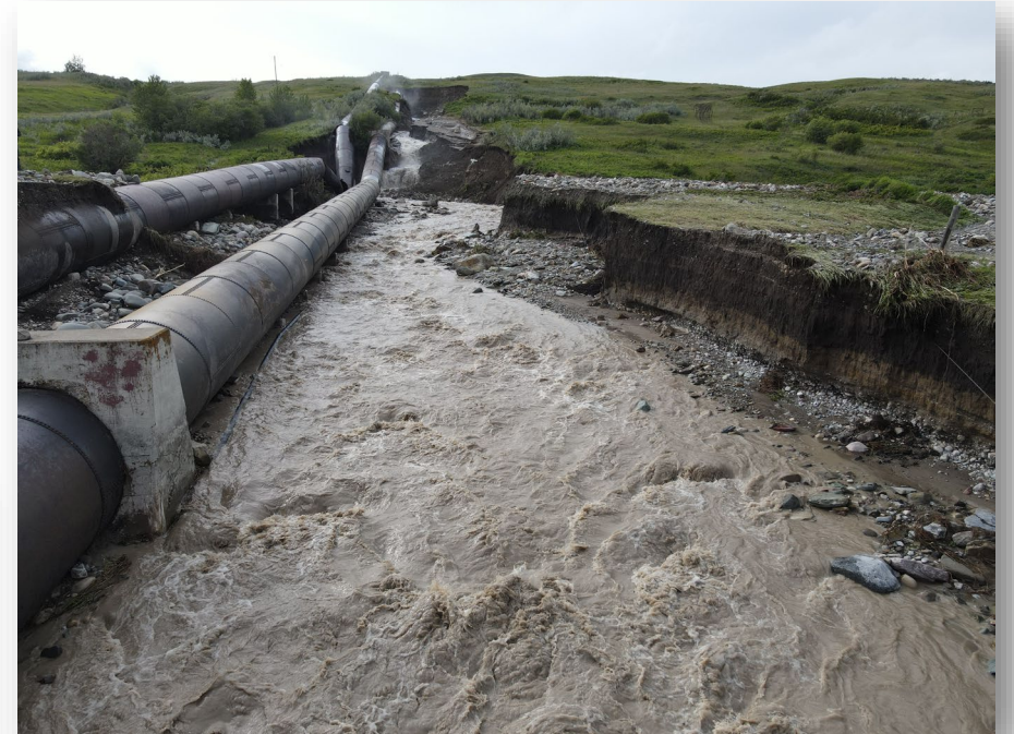
St. Mary Siphon's two 90-inch siphon pipes, which transport St. Mary Canal water across the St. Mary Valley, failed while diverting approximately 600 cfs.
