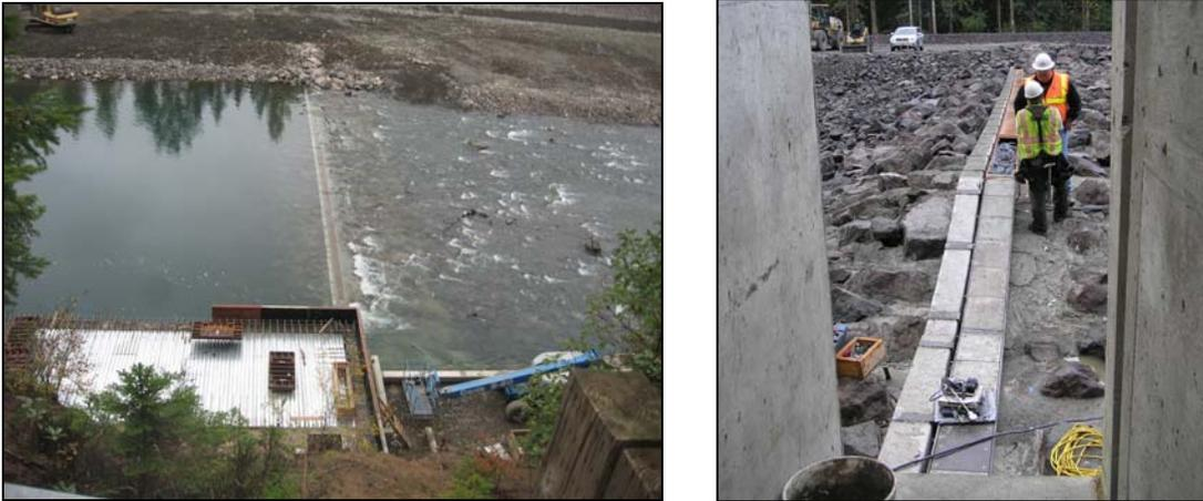
**Figure 3. New diversion weir (river km 5.6) constructed across the Elwha River in October 2008. The picture on the right shows the low flow notch during construction. Flow direction in both figures is from left to right.**
