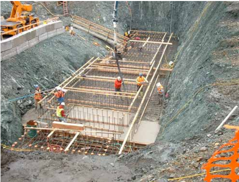
Placing slab no. PP-S-2. 2/20/07
