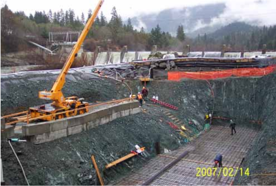
Re-steel installation.
