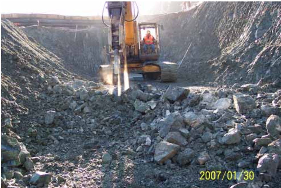
Greenstone being broken with a hydraulic ram.
