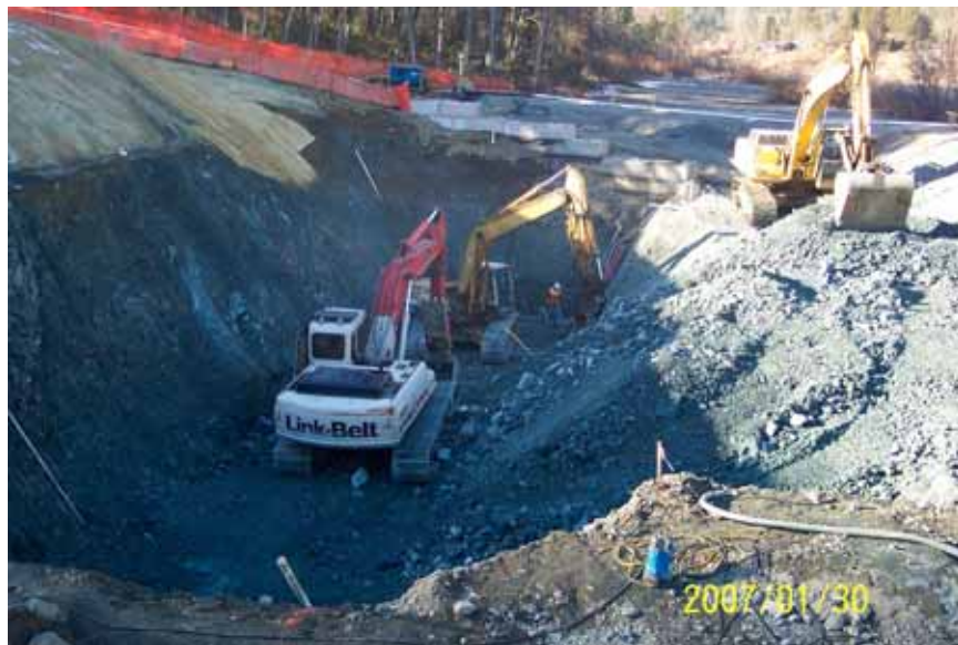
Pumping Plant excavation continuing.
