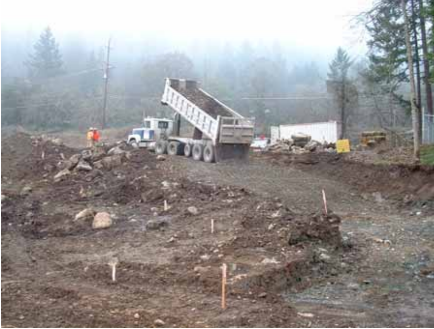
View of intake structure access road construction. 12/6/06
