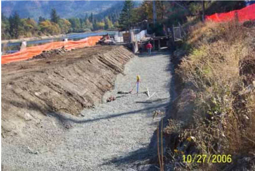
Grading for pipe arch in gravity canal.
