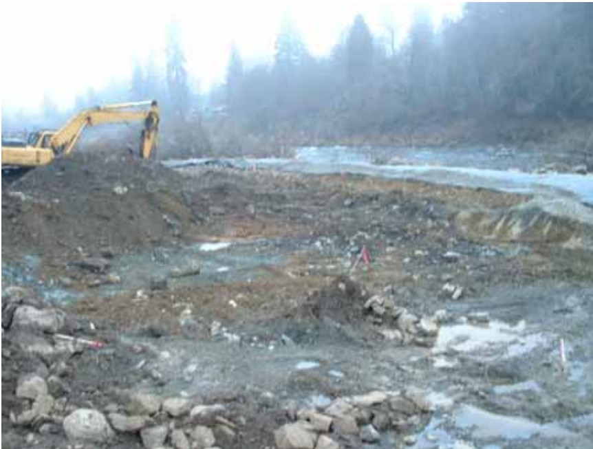
View of pumping plant excavation. 12/6/06
