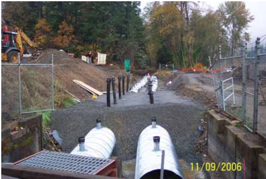
View of pipe arch and vents installed in the gravity canal
