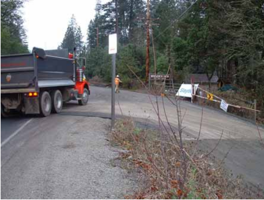
View of new driveway. 12/7/06
