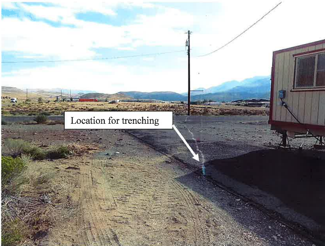
Photo 2. Facing east towards existing power pole
