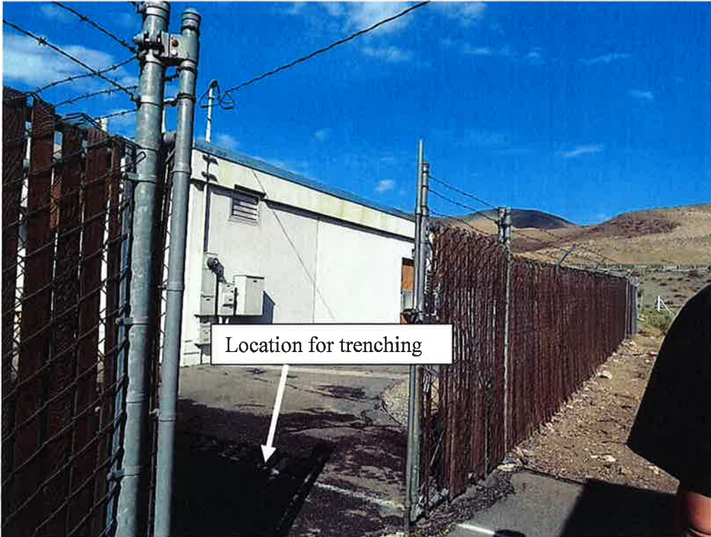
Photo 1. Facing west towards AT&T/Nevada Bell telecommunication site
