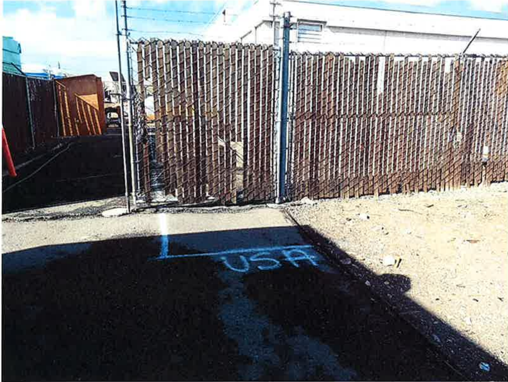
Photo 3. Facing south-southwest towards the existing telecommunications site
