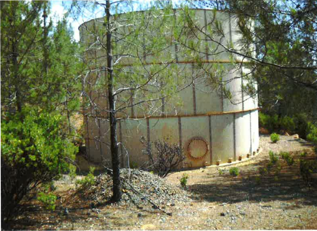
0.15 MG storage tank (32-feet wide) to be replaced with a 0.50 MG steel tank (60 feet wide). (Image from ENPLAN 2013).
