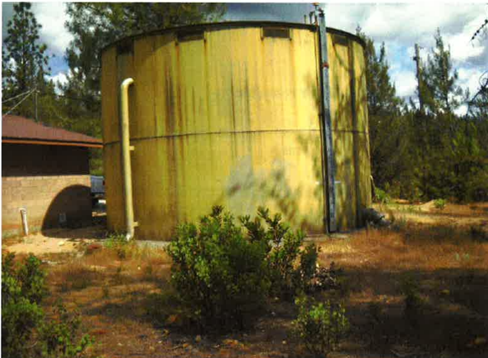
0.05 MG storage tank to be converted to a backwash tank (image from ENPLAN 2013)
