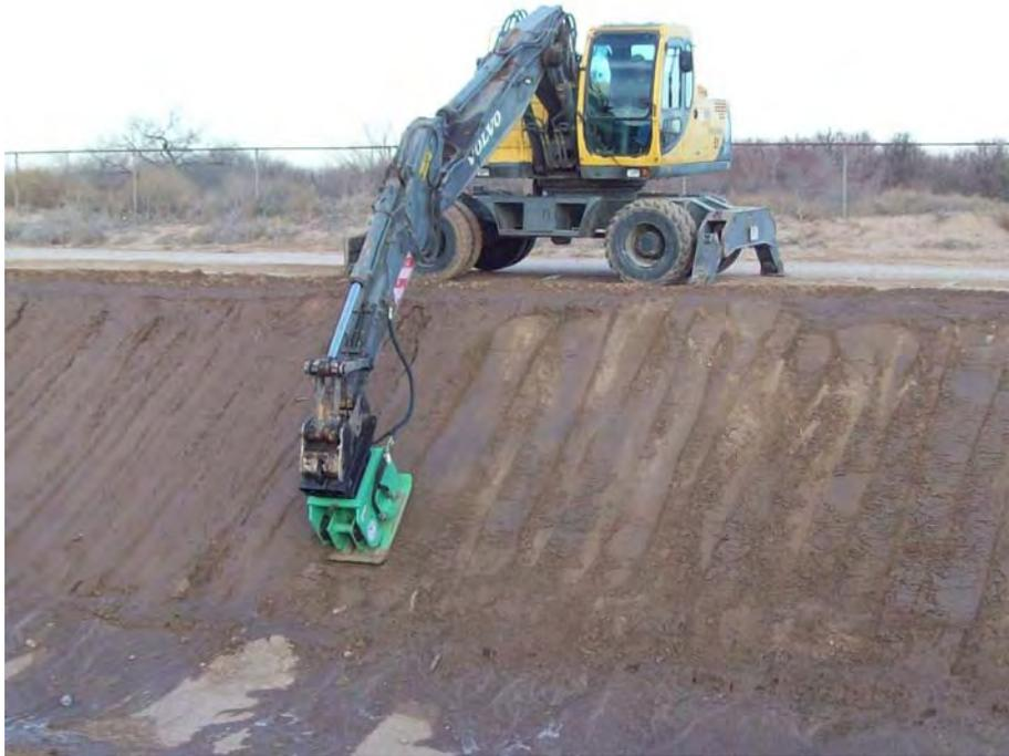
Figure 5 - Vibratory compactor canal wall stabilization. Source: AW Blair Engineering (2011)
