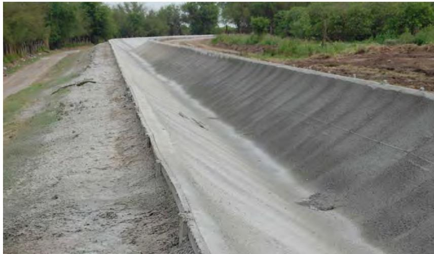
Figure 4 - Fiber-reinforced shotcrete application. Source: AW Blair Engineering (2011)
