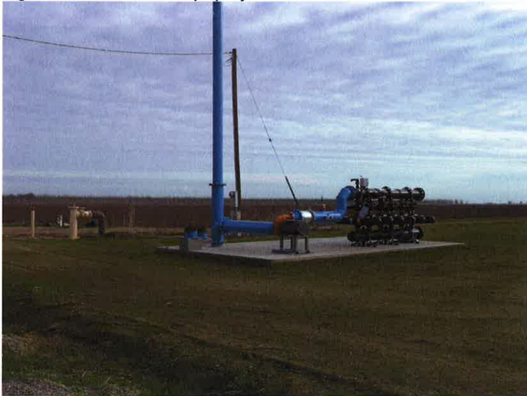
Attachment 3. Existing pump station where water would be made available to irrigation lines to the annexed property.
