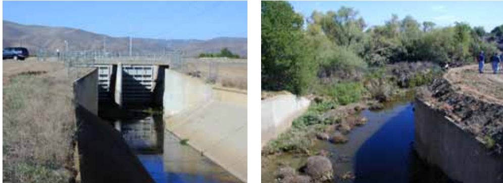
Figure 3-3. Westley Wasteway at DMC (a) and at Bypass to Private Refuge (b)
