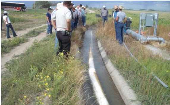
SDSU innovative suction filter for center pivot pump near Oral, SD. Flood irrigation to center pivot conversion.
