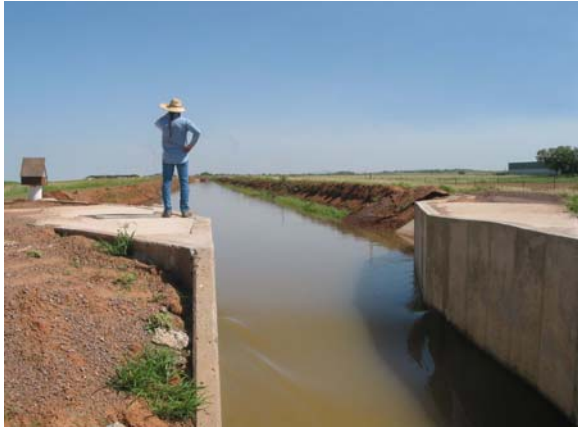
Altus Canal flume constructed by District in 2004
