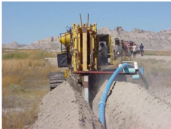
Installing water line on the Mini Wiconi Rural-Water System, SD
